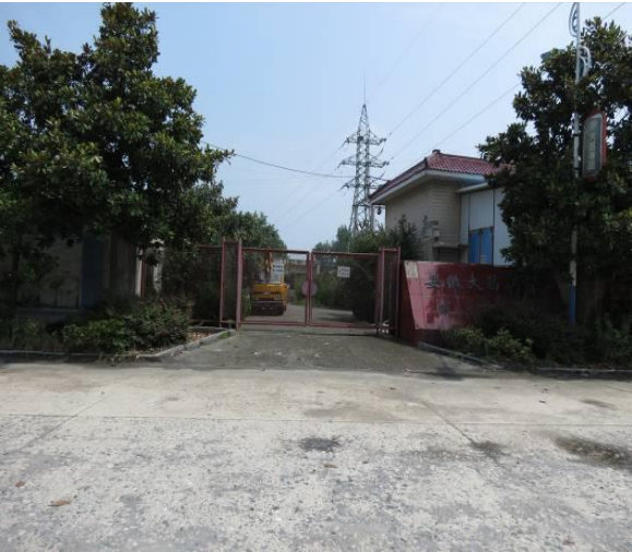
3-25(续) 2#变电站现状
